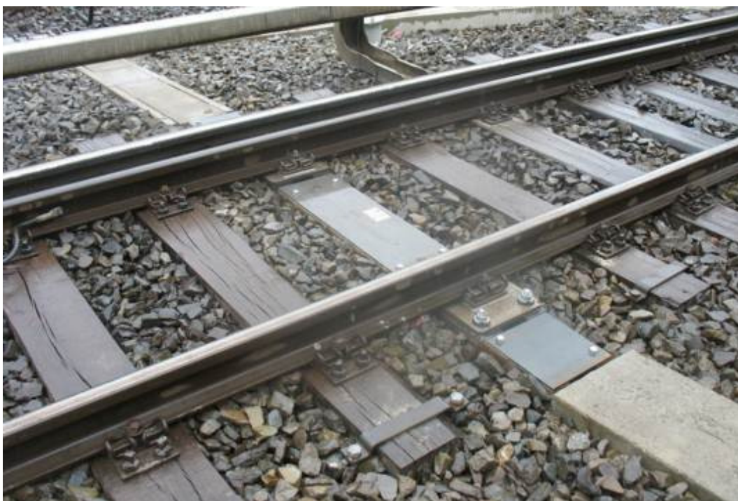
After: tamped track, cable passing inside Schwihag hollow sleeper
