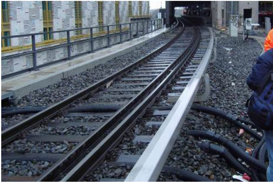
After: tamped track, cable passing inside Schwihag hollow sleeper
